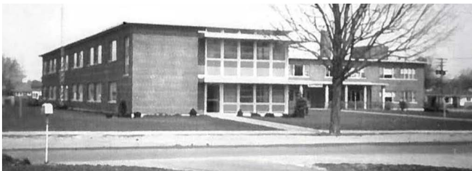
Photo following the completion of the West Wing addition in 1961.
