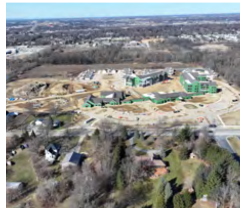
Progress on The Farmstead
